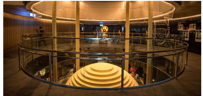
A visitors' gallery provides a close up view of the Taipei 101 TMD in operation.
