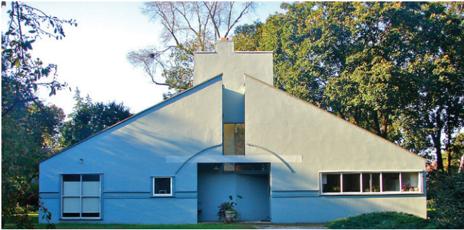
Vanna Venturi House. Note the unexpected scale and placement of windows, a split gable, unconventional configuration of the front entrance and the suggestion (only) of a curved porch roof.
